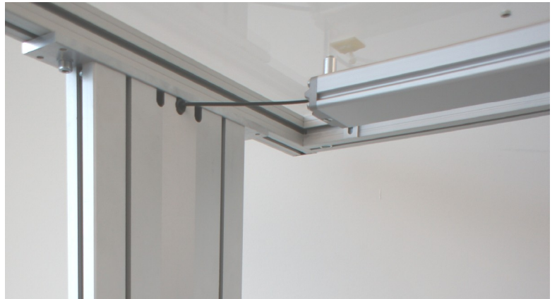
Connection hose from cylinder to pump
