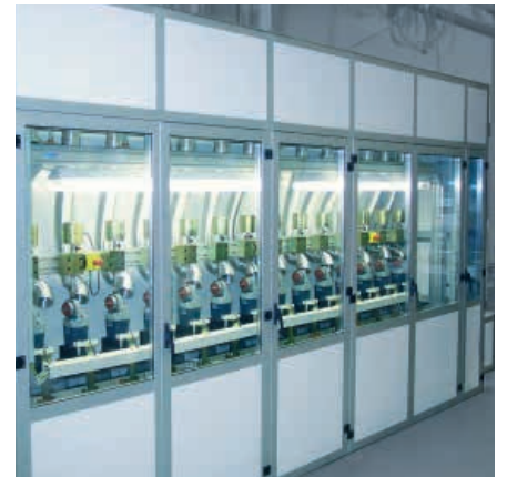
Protective cabinet and noise protection
